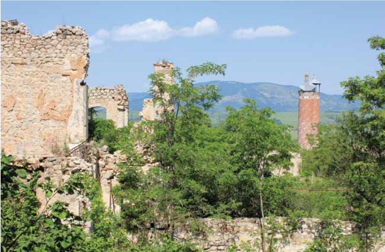
Derelect buildings dominate Shusha, Nagorny Karabakh's only former Azeri-majority town.
